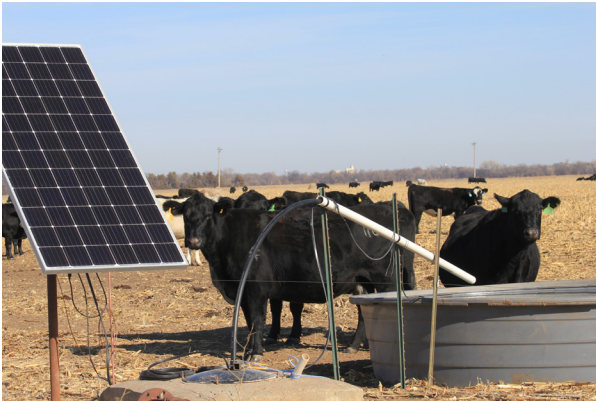
Photo 9. Solar pumping system with well at edge of crop field.
