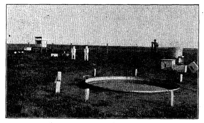
PLATE 2. The weather instrument used at the Hays Branch Experiment Station to determine rainfall and evaporation.
