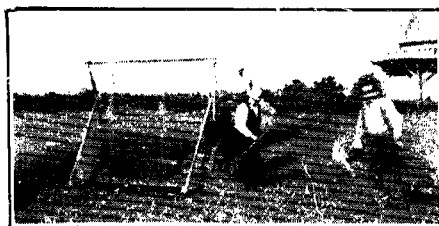
FIG. 27.—The hand rake reaper was first used for harvesting wheat about 1830. It was the forerunner of the modern self-binder.
