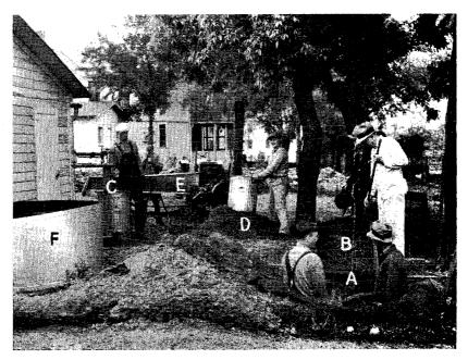
FIGURE 2.—Filling a pit silo with grass silage. The silo is represented by (A); the mixing box (B); the scales for weighing (C); the finely-chopped grass (D); the ensilage cutter (E); and the superstructure (F).
