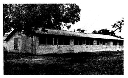
FIGURE 5.—The house where the experiments with laying birds were conducted. It was divided into four lots each 20 feet square. Note unevenspan, metal-covered roof. The open front was equipped with muslin curtains which could be closed one third, two thirds, or fully closed as shown in the second lot from the right. A 1-inch wire mesh ceiling was covered with 12 inches of straw. Rear ventilators were used during the summer.
