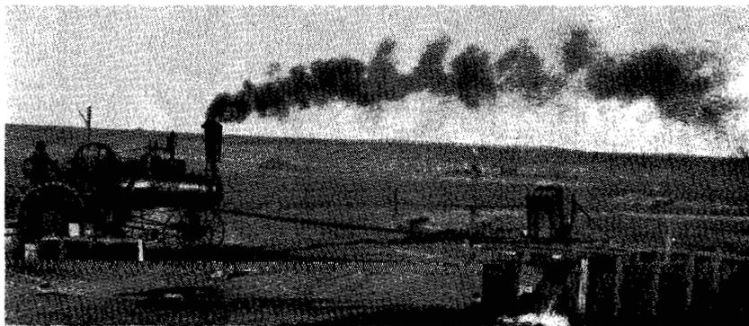
Fig. 29.—Irrigation investigations were started in 1903 in cooperation with the U.S.D.A. A Knowles centrifugal pump was operated with a J. I. Case steam engine.
