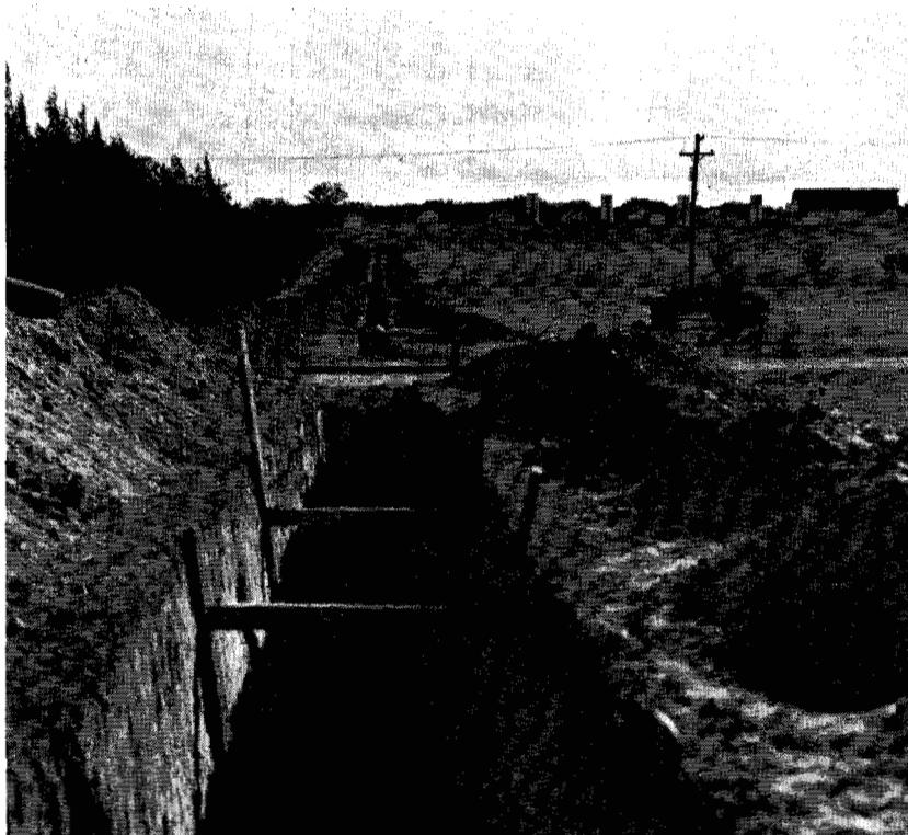
Fig. 22.—Sewer line east from flush tank. When the city of Hays installed a new sewage disposal plant in 1935 permission was granted for its installation on Station land, with the agreement that the Station could connect its sewer to the city's.
