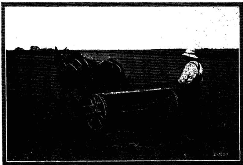
Fig. 9.--An alfalfa drill. A good drill insures an even distribution of the seed and a uniform depth of covering.
