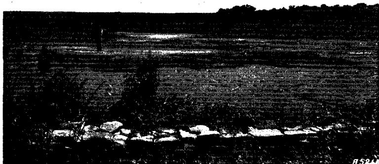
FIG. 9.—A rock dam across a broad ditch has caused a large amount of soil to be deposited. This has tended to level the field somewhat and has prevented the loss of a large amount of fertile soil.
