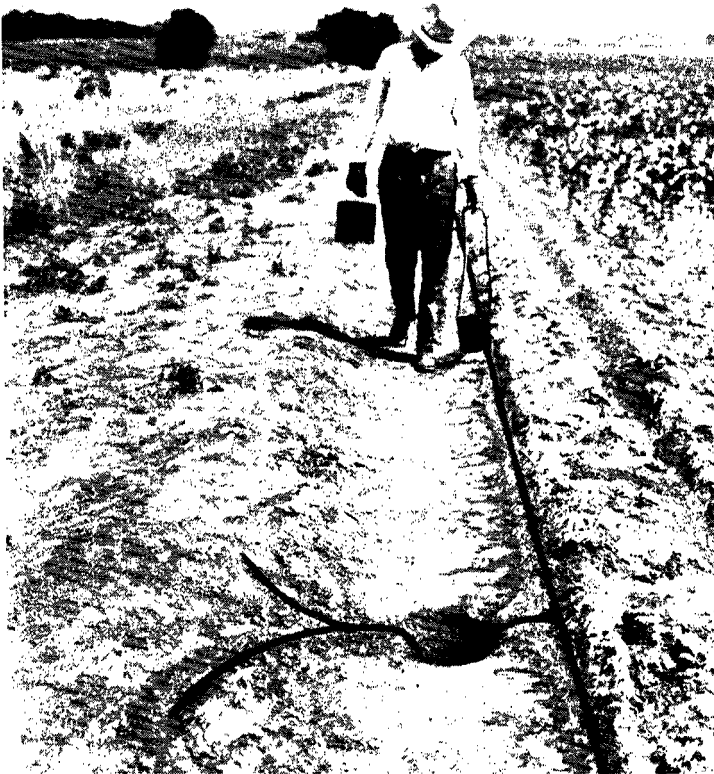
FIG. 17.—A creosote-post-hole barrier showing method of pouring creosote with a long-handled gallon bucket.
