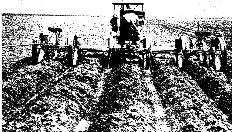
FIG. 5.—Nosing out old furrows with disks attached to the runners of two-row planters. This permits the sorghum seed to be dropped in a warm, mellow seed bed.
