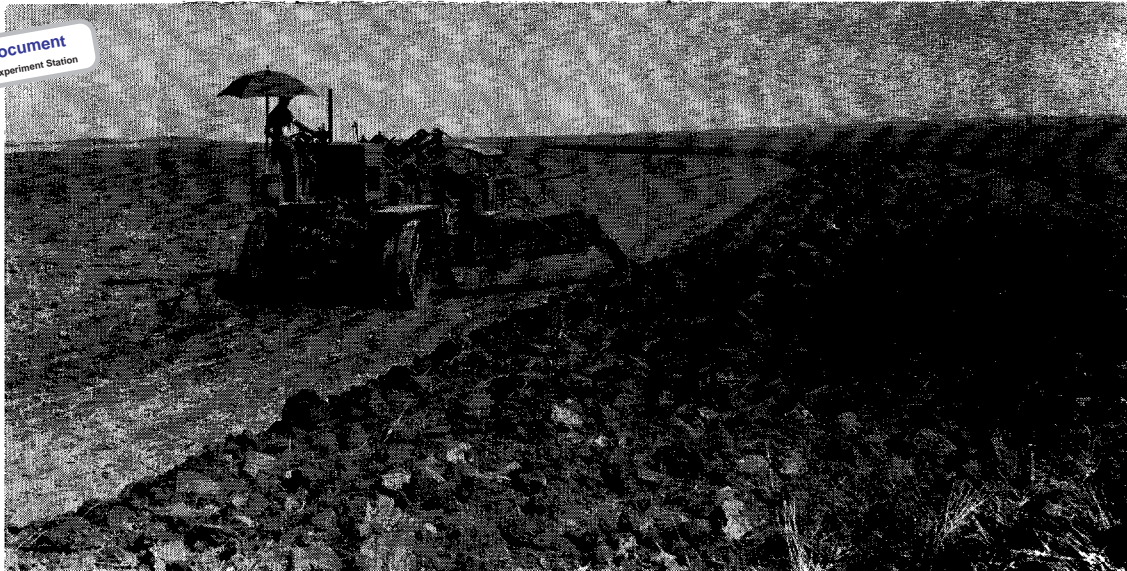
Fig. 71.—An elevating grader was used to construct some 10 miles of terraces to conserve water and to control soil erosion on the cultivated land of the Station.
