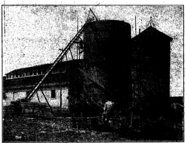
Fig. 3.—Some silo-filling equipment. Notice the silage cutter with open carrier
