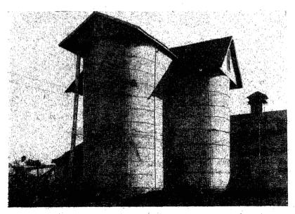
Fig. 1.—Filling a silo with sorghum. The cut material is forced up through the pipe by a blower
