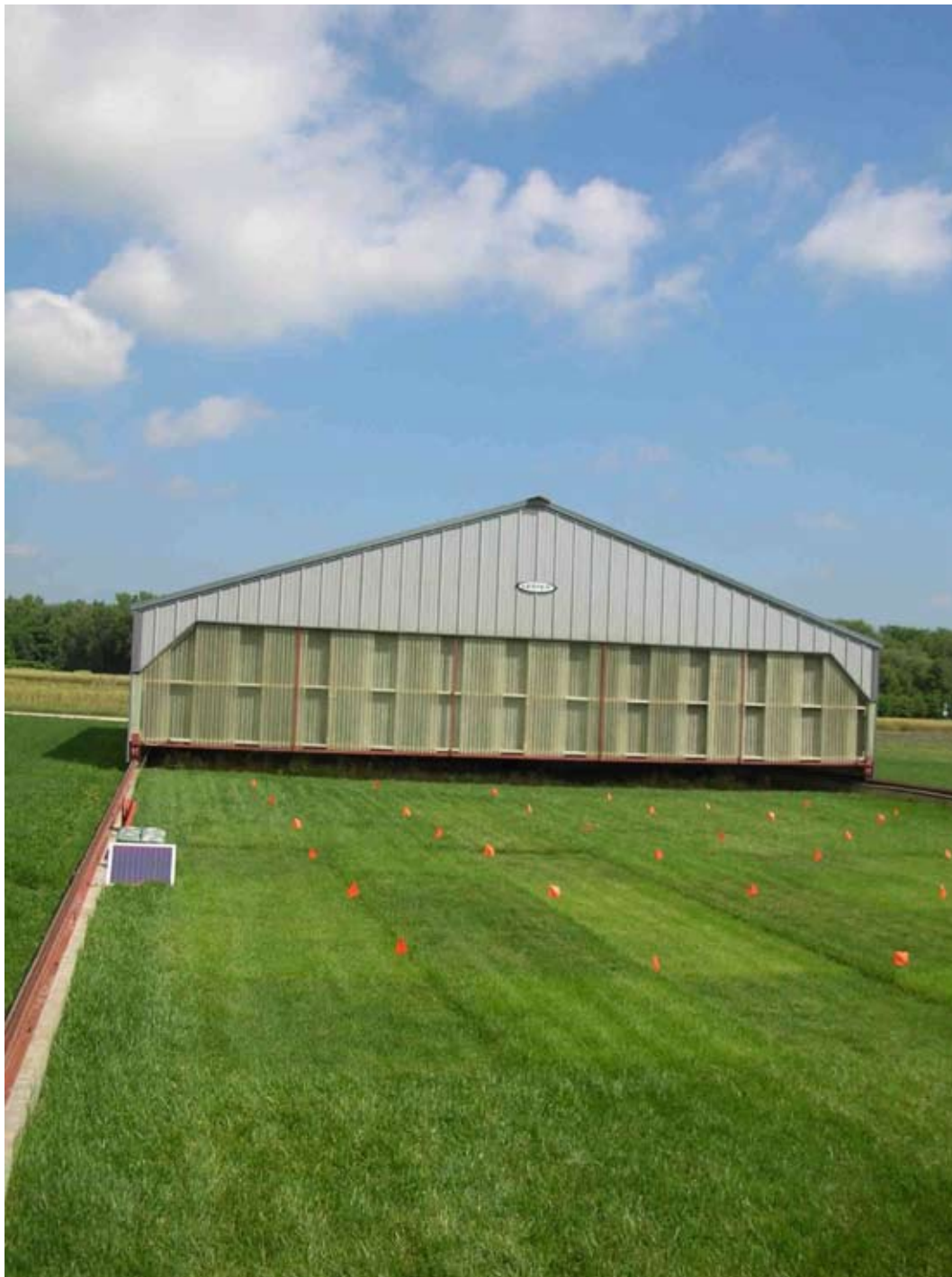
Figure 1. Rainout shelter (180 m 2 ) at Rocky Ford Turfgrass Research Center near Manhattan, KS. The rainout shelter automatically moved over plots (on tracks) when rainfall began, then retracted one hour after rainfall ended.
