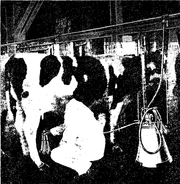
No. 62.—Operator holding teat cups turned back ready to attach.
