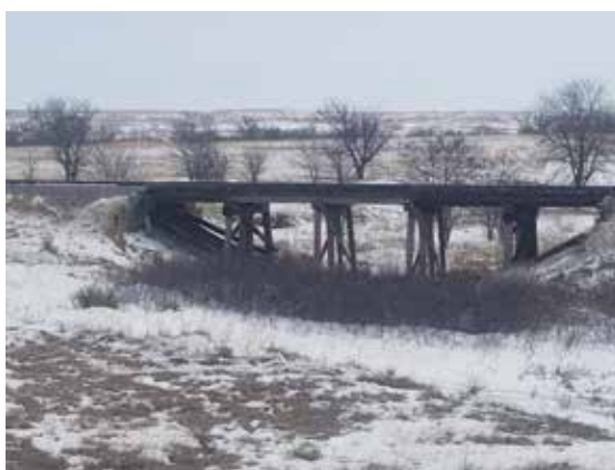
Figure 11. Vegetation around wooden bridges can be a serious fire hazard. Photo: Frannie Miller
