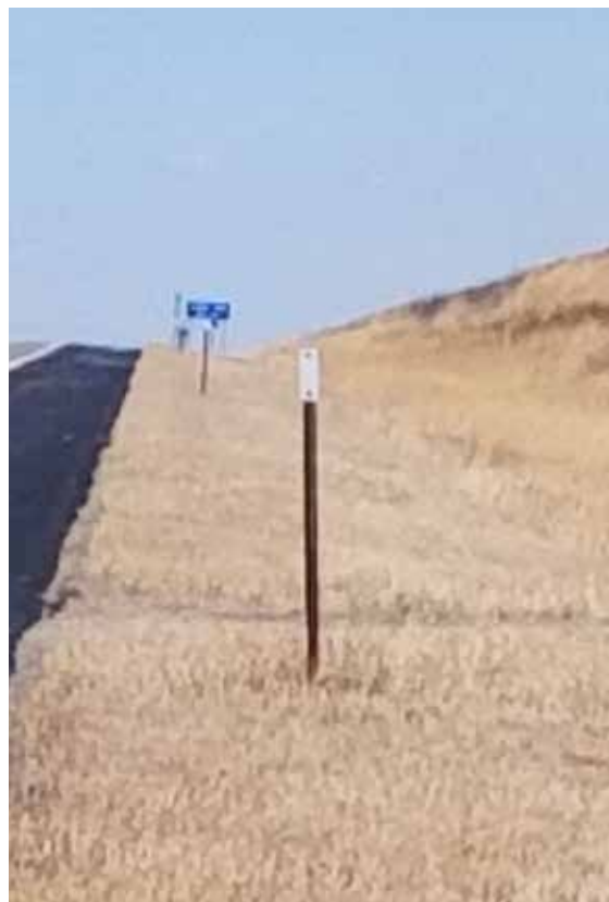
Figure 3. Total vegetation control around delineator posts facilitates mowing. Photo credit: Frannie Miller
