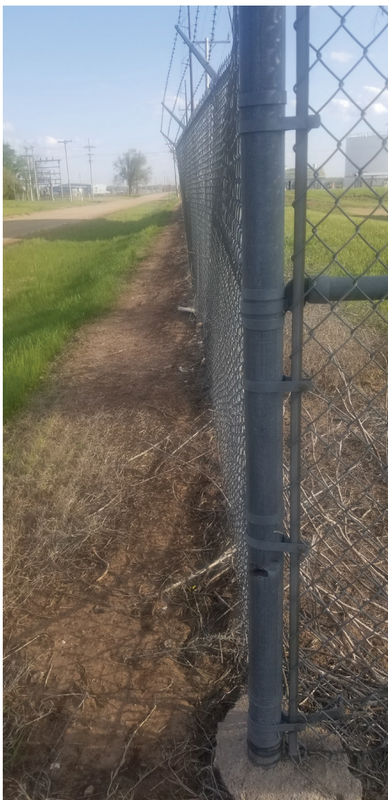
Figure 4. Weed control under fences reduces maintenance costs. Photo credit: Frannie Miller
