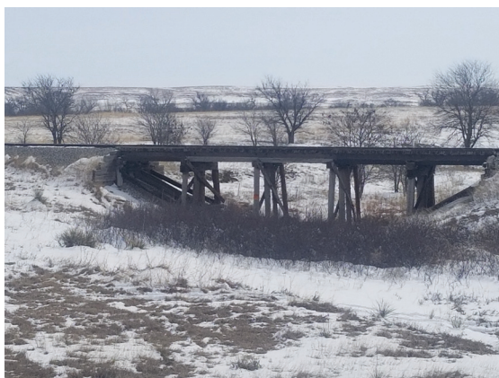
Figure 11. Vegetation around wooden bridges can be a serious fire hazard. Photo: Frannie Miller
